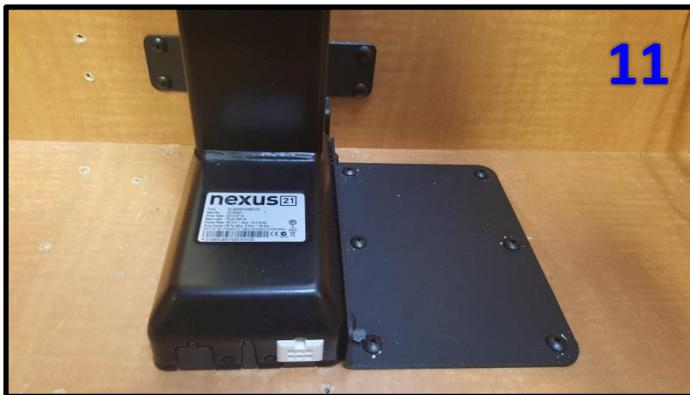
**Step 11:** Center the Lift horizontally in your cabinet and mount the Lower Column Support and Base Plate for each column to the cabinet using (20) 10 x 3/4" THWS Screws.
