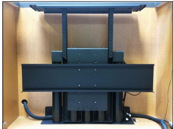
**Step 24: Attach the Lower Column Braces to the cabinet.**
